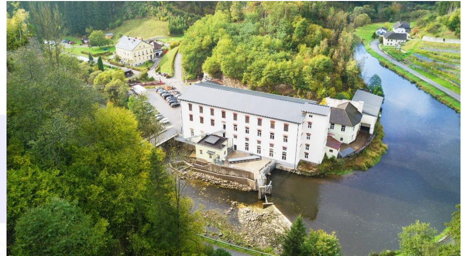
Foto Provided by WWS Wasserkraft GmbH
