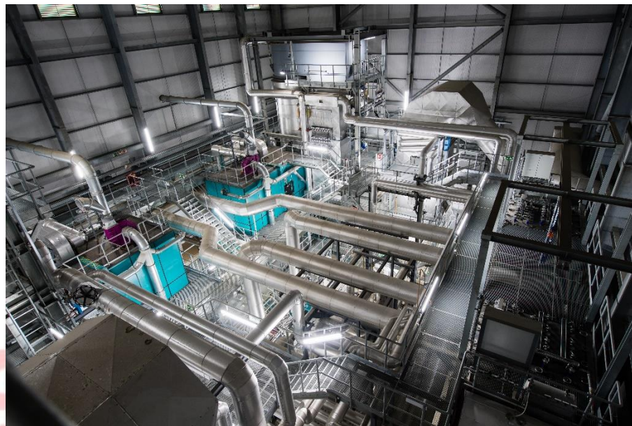
View of a 2 x 10,000 kW combined heat and power plant (3,000 kWel) in Wales Credit: Polytechnik GmbH
