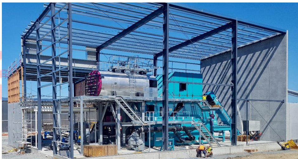
Installation of a 5,000 kW biomass combustion plant with hydraulic moving grate Credit: Polytechnik GmbH
