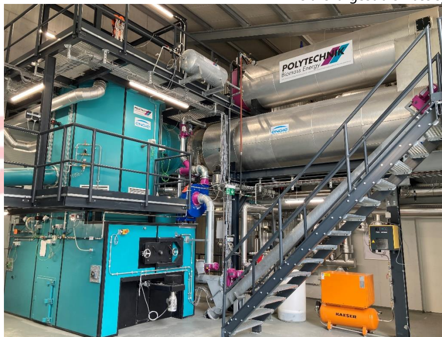
1.000 kW Poly-H.E.L.D. - novel combustion technology (high efficiency - low dust) Credit: Polytechnik GmbH
